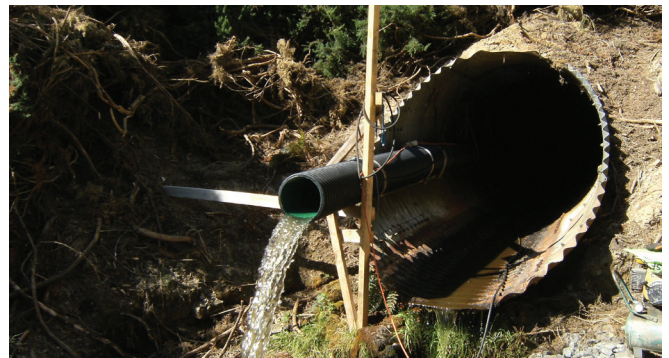
EUROFLO® inside a damaged pipe
