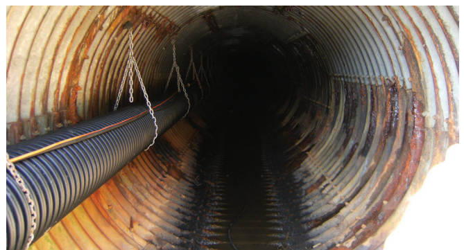
Fixing EUROFLO® inside a damaged pipe
